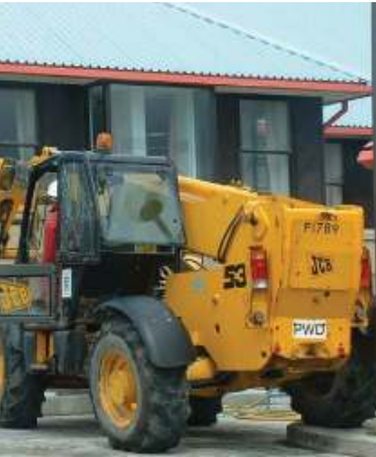
Delivery of the shell of its new isolation ward. The isolation ward will become an elderly care ward.
