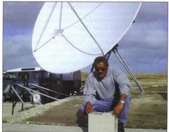
British Forces Broadcasting Services engineer Albert Quatre re-aligns the satellite disk at Mount Pleasant Airport after a gale. It had been shifted only by millimetres, but this was enough to interrupt the incoming TV signals. KTV transmissions in Stanley were not affected.
