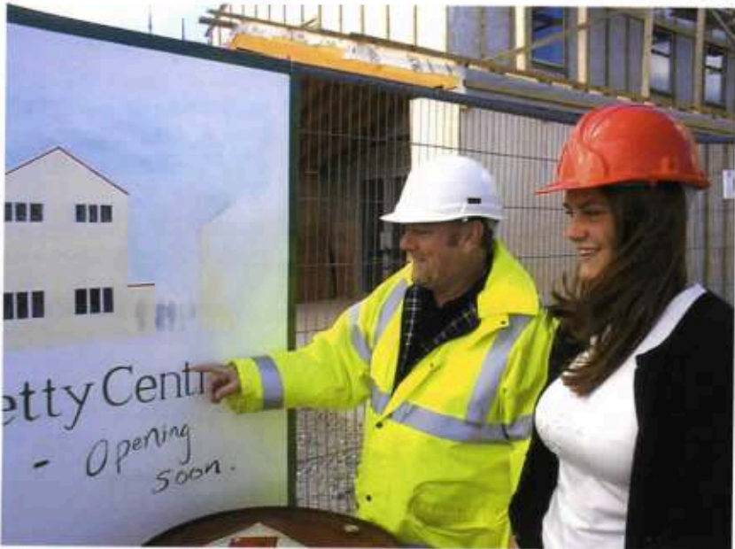
Miss Emma Jane McAdam and Mr. Mark Thwain at the visitor centre construction site - where many of her ideas will be incorporated.
