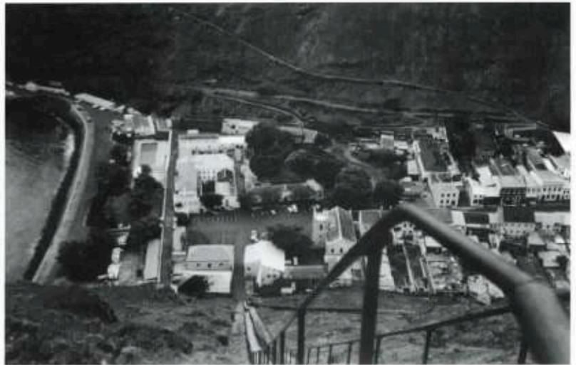
Jamestown photographed from beside Jacobs Ladder, the famous 699 step stairway to the fortifications above the town.
