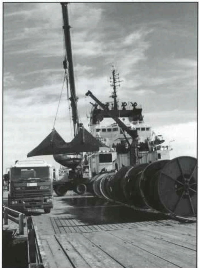
One of the huge anchors that attach the floating drilling platform to the sea bed being unloaded in Stanley. Photo: Norman Clark.
