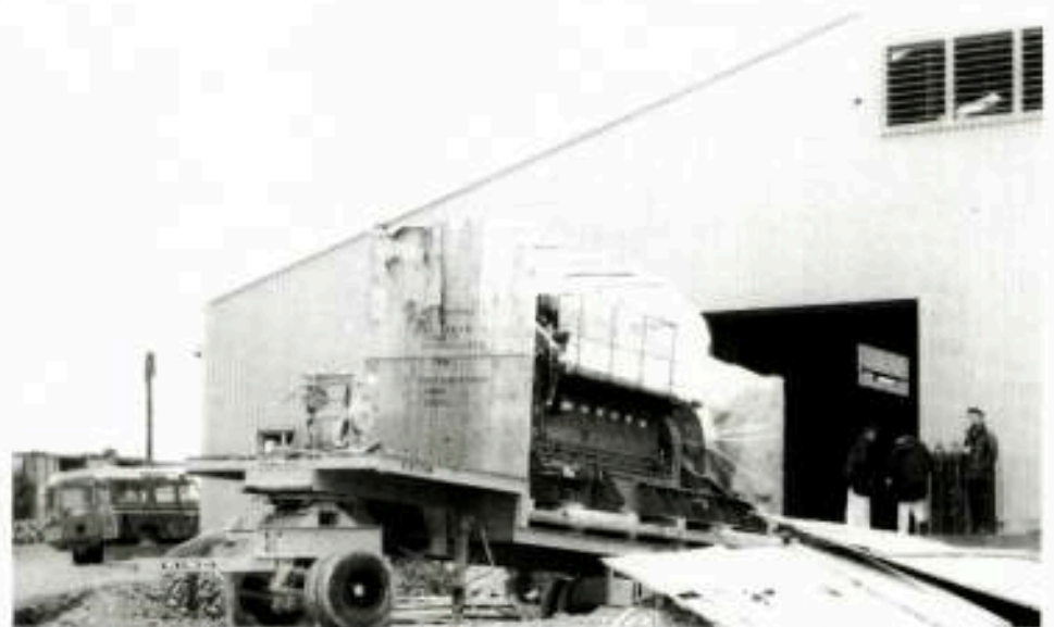
New Generator Arriving at Stanley Power Station (Photo: R. N. Spafford)
