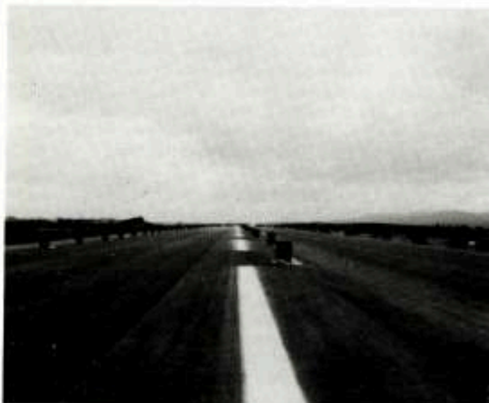
Awaiting the arrival of the first Jumbo, Main Runway, Mount Pleasant Airport, Falkland Islands (Photo: R. N. Spafford)
