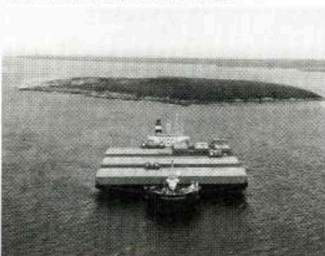
Final section of the Flexiport carried on the Dyvi Teal in Port William is moved towards Stanley Harbour. (Crown copyright: photo by Forces Photo Section, Falkland Islands.)
