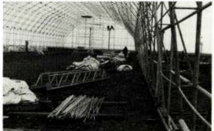
The Rubb Building under construction, Mount Pleasant
