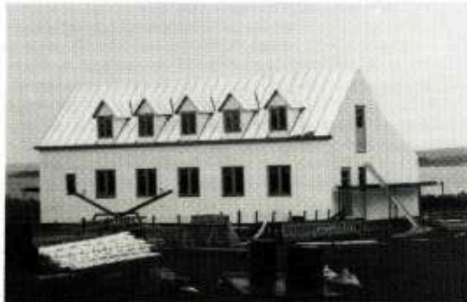
The new school at Goose Green nearing completion
